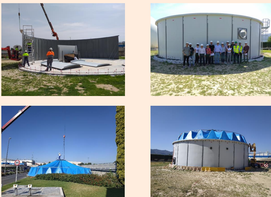
Figure 8. Views of the elutriation tank assembly
